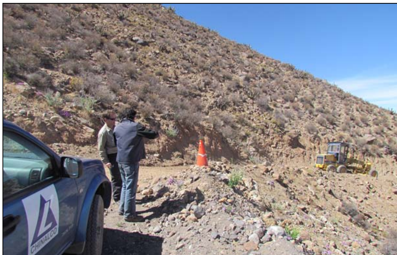
Road cleaning to the Candelabro Prospect – October 2011.
